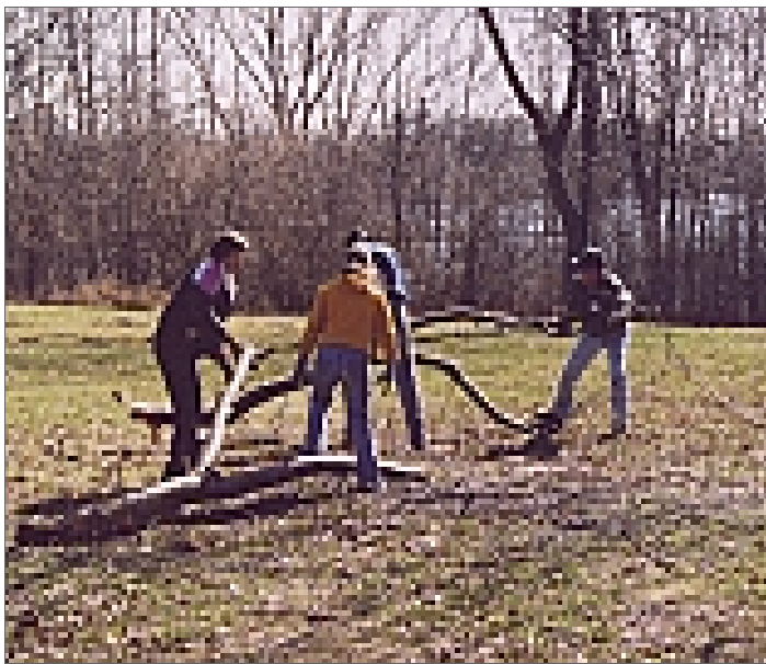
Crews work on the beach areas.
