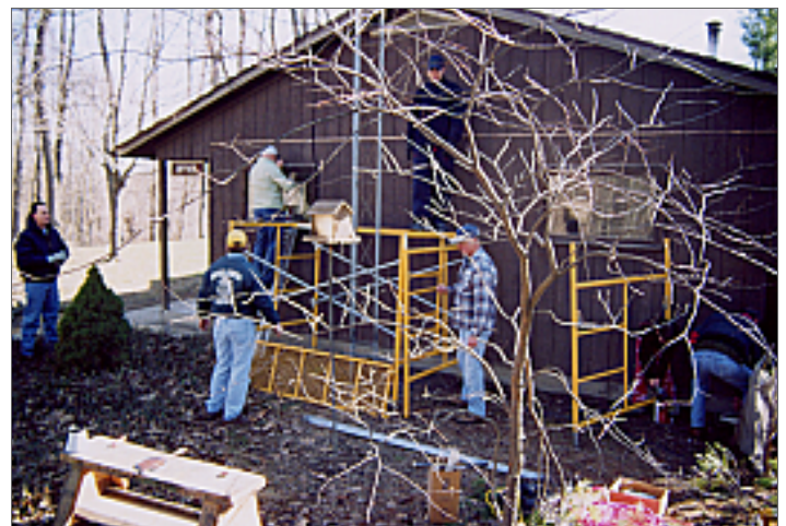
Park Headquarters getting a coat of paint.
