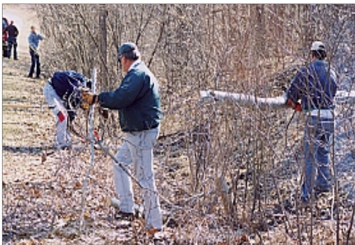
Clearing the main road into the Beach.
